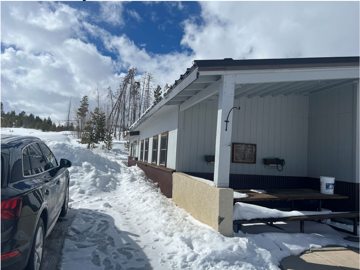
Image 1 District Office Building Roof Profile
